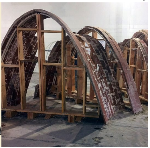
the tiles are then sandwiched together to form the outer 'shell' structure whilst the interior will be
